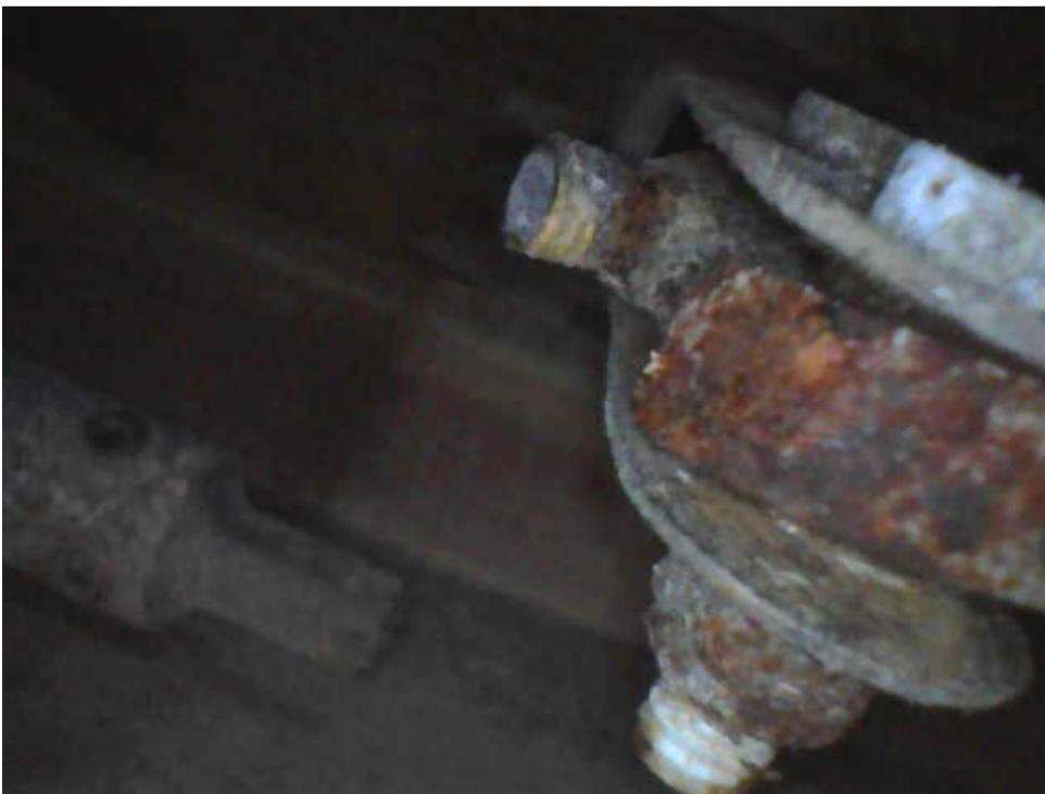
Picture 1 Corroded and fractured push rod rod end inside a wing.
